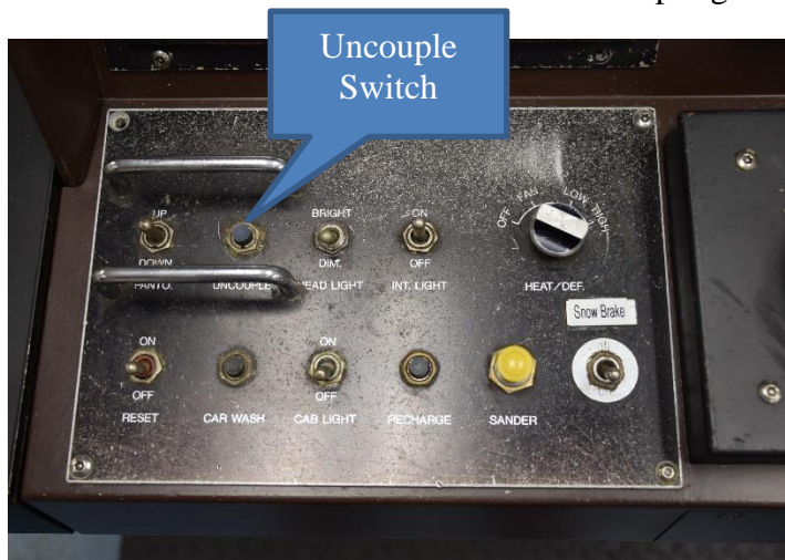
Figure 3.18 Uncouple Switch, Courtesy of GCRTA
