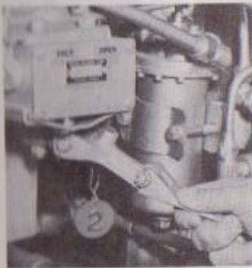
Coil Blowdown Valve-2 Fig. 6-8
