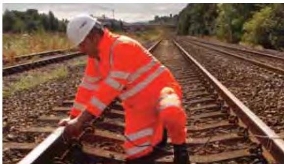
Using a track-circuit operating clip
