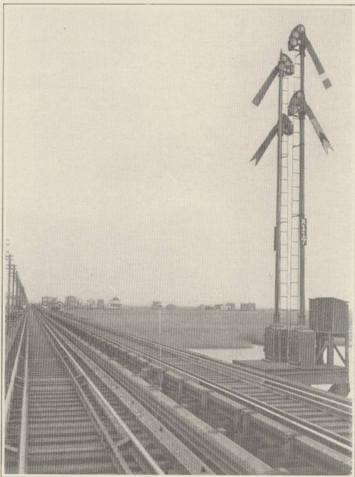
SIGNAL, LOCATION ON TRESTLE.
