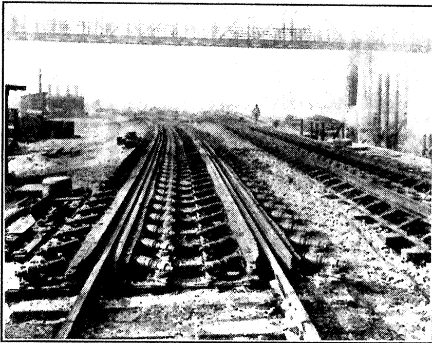
Fig. 16. Electro-Pneumatic Retarder, Boston Type.
