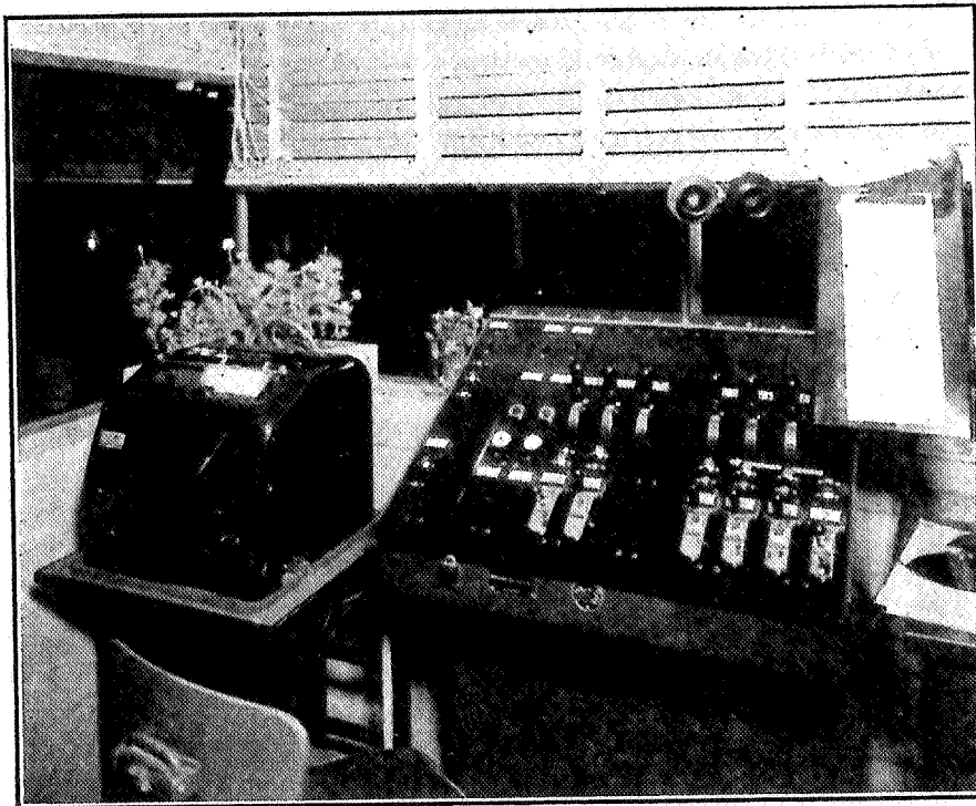
Fig. 40. Electric Control Machine in Junction Switch Tower.
