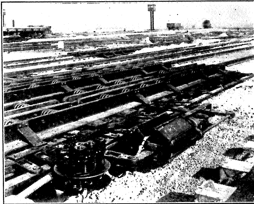
Fig. 10. Electro-Pneumatic Retarder, Markham Type.
