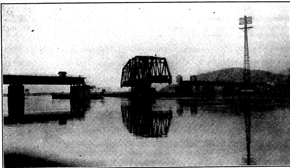
Fig. 36. Center Pivot Drawbridge.
