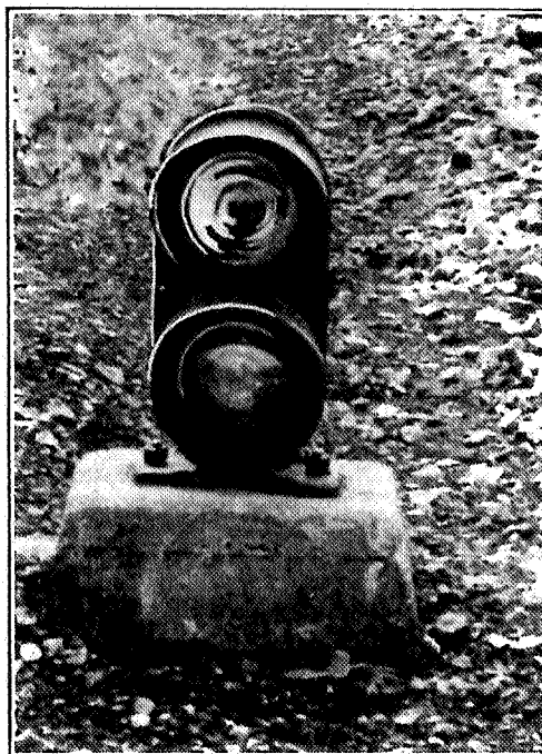
Fig. 10. Style N-2, Color Light Signal.
