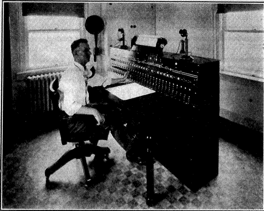
Centralized Traffic Control Machine on New York Central Railroad.
