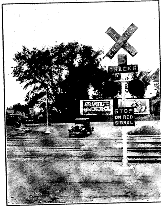
Highway Grade Crossing Signal Installation on Erie Railroad.
