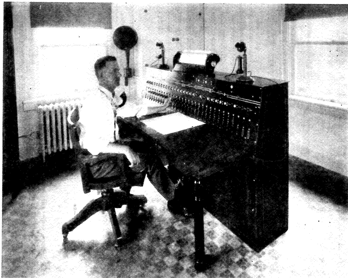
The control machine for the first installation of the G.R.S. dispatching system (C.T.C.) between Stanley and Berwick, Ohio, on the New York Central R.R. (1927)
