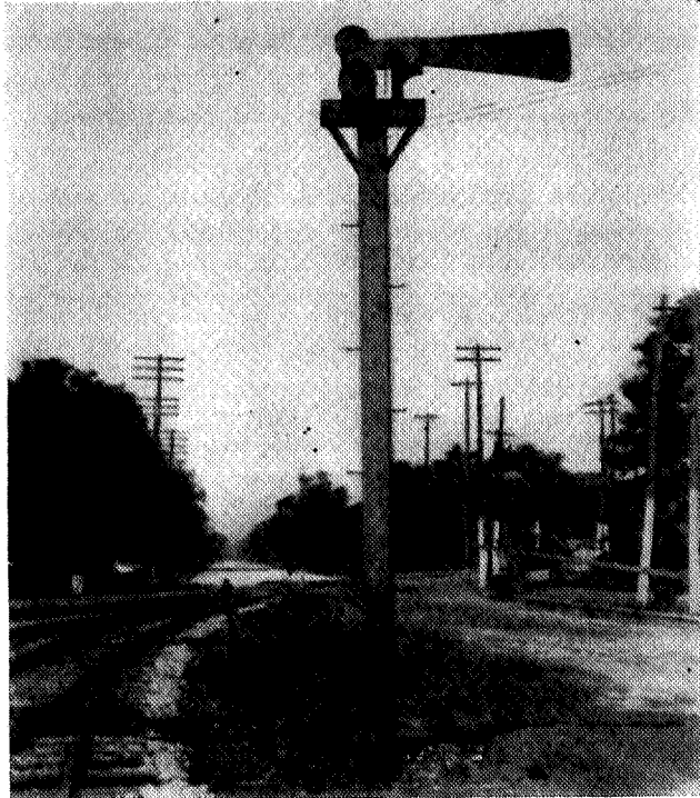
This Cox type of station signal, a three-position, upper-quadrant semaphore, was installed on the Kentucky & Indiana R.R. in 1887.
