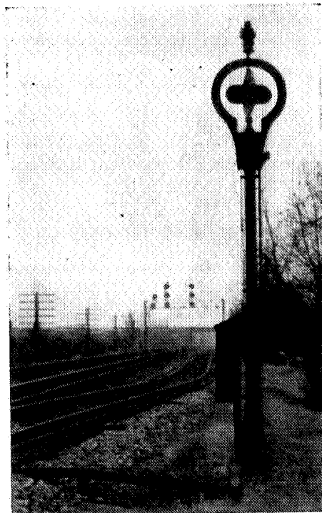
Exposed disc clockwork type signal on the New York & New England R.R. (1882).
