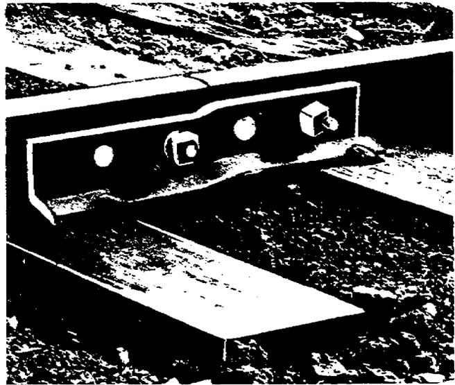
Compromise bars compensate for differences in web thickness, head width and depth, height, and location of boltholes. A pair of compromise joints holds the smaller rail so that its top and gage side meet those of the heavier rail. When compromise joints are ordered, the two rail weights and sections and the direction of the joints are specified. Compromise splices are common in theaters because they allow the use of any rail regardless of its section.
