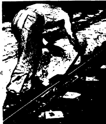
necessary before the next routine maintenance period. How tight the bolts are to be drawn initially should be within the range set--in excess of 10, 000 pounds per bolt is specified on some roads.
