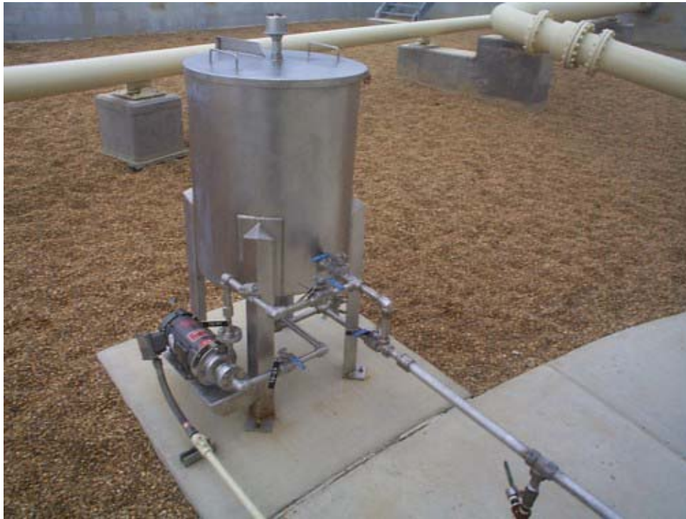
Figure 7.2. Water Draw-Off System.
