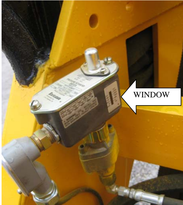
Close Pressure Control Switch (Located in front corner of LH Walkway)
