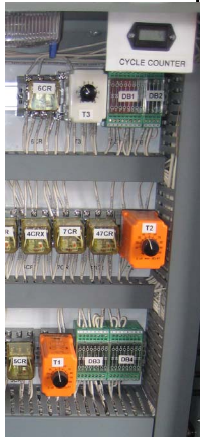
Figure 3. Cab Controls and Indicators Inside Main Control Panel (Right Cab Wall Behind Operator)
