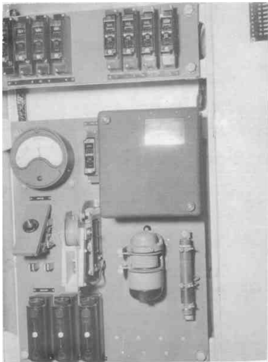
LOW TENSION PANEL : NO. 2 END.
