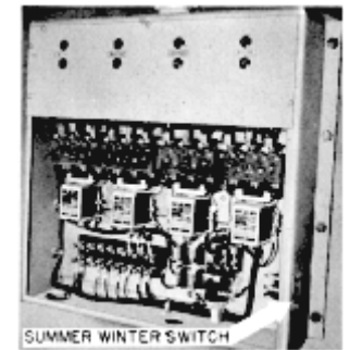
AC Contactors Fig. 4-1
