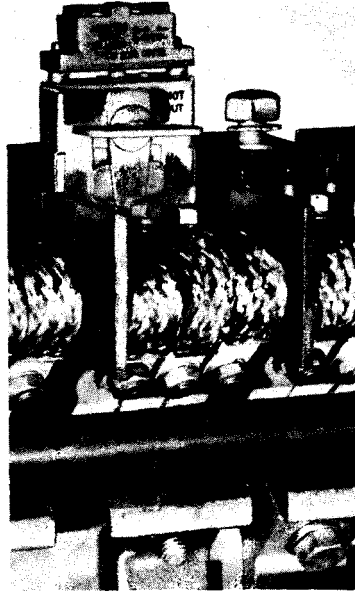
Motor Lockout Switch Fig. 2-16
