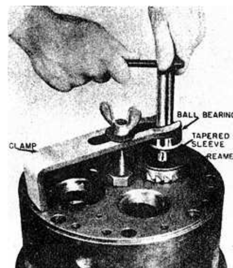
Cleaning Valve Guide Fig. 2-20
